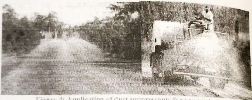
Figure 4: Application of dust suppressants for unpaved roads
